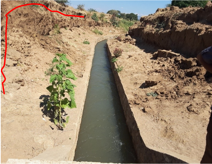
Photo 6.3: Irrigation canal for Mwenda-Mtitu irrigation Irrigation Scheme that is susceptible to be filled with landfalls as it was taken by auditors on 21 st July 2018
